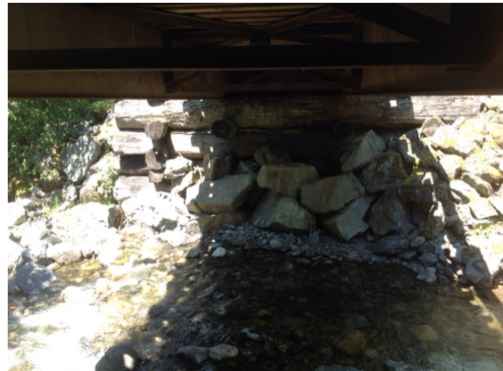
Right Bank Abutment when facing downstream
