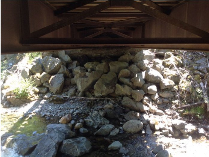
Left Bank Abutment when facing downstream
